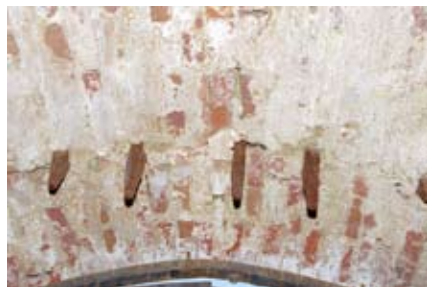
Герса, вмурованная в свод ворот при ремонте XIX в. A porcellis immured into the gate arch during repairing works in the XIX century
