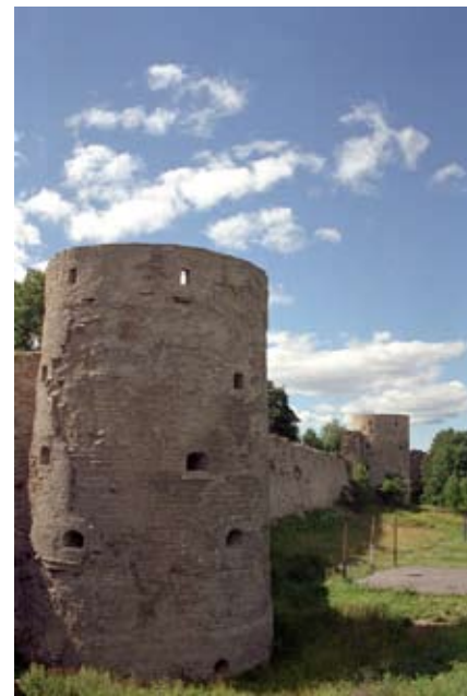
Северная стена крепости Northern wall of the fortress
